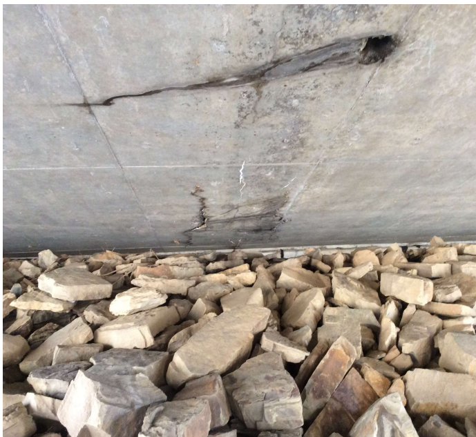
PHOTO 3 Description Typ. Delam & Cracking in Soffit under Long Cracks in Deck.
