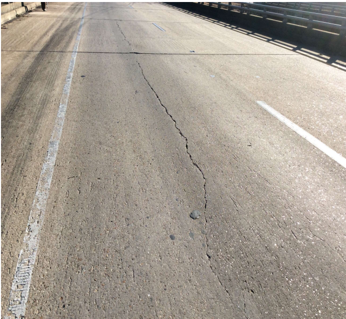
PHOTO 1 Description Typ Long Cracking in all .Spans
