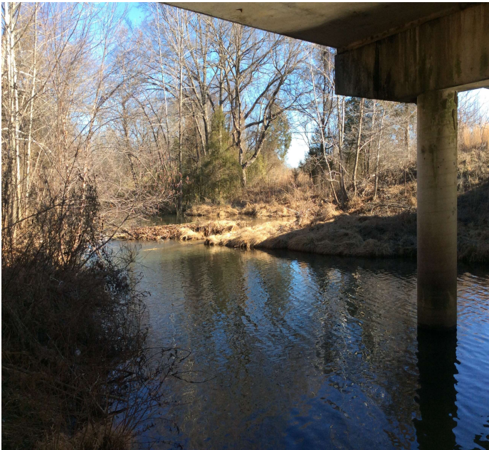
PHOTO 1 Description Brush, Veg. & Silt in Channel Blocking Flow on Lt. (Up) Side.
