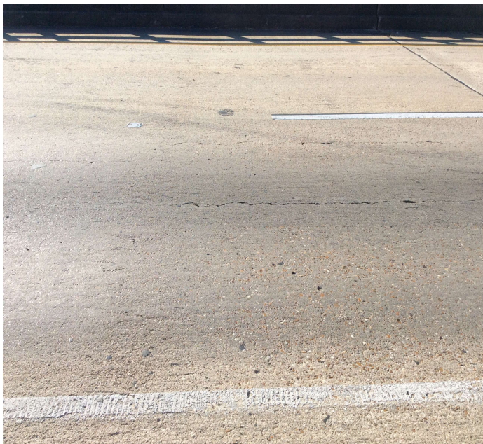
PHOTO 4 Description Typ. Cracking in Deck.
