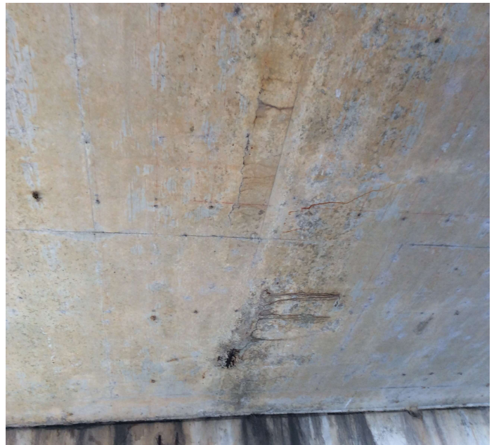
PHOTO 2 Description Cracking & Spalling W / Rebar Exposed in Soffit unde Long Cracks in Deck.
